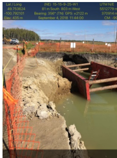
Sept 4/18 Cracked stairway of entry of excavation Notified Enbridge safety of unstable ground Notice cracks bottom of picture unstable walls, cave in ahead of trench box
