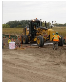
Sept 6/17 823 + 253.0 Photo taken facing north west Grader being pressure washed
