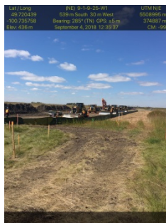
Sept 4/18 SSKP 829+253 Biosecurity Management cleaning station Dozers getting soil removed and debris Also mist disinfecting any piece that comes into contact with ground
