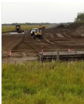
Sept 8/18 KP-830+923 D8-dozer stripping soil Bob-cat moving mats
