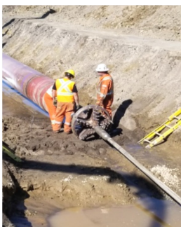
Sept 7/18 KP- 826+745.0 Workers getting ready to start the stringing Photo taken facing east
