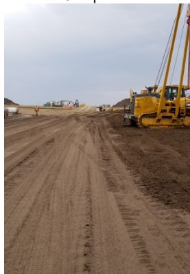
Sept 8/18 KP-826+650.0 Photo taken facing North. Ream and pull the enbridge corridor bore. South fo SF #21
