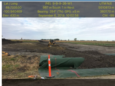
Sept 6/18 SSKP 808+600 Stripping Kick-off to Rd #1 Dozer building road approach Flume pipe under geo tec, facing west Flume pipe used to let water through
