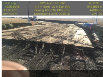
Sept 4/18 Conditions on ROW muddy from rain At location noticed a knocked down sign Mats to step to access ROW Facing East with low bed truck in background
