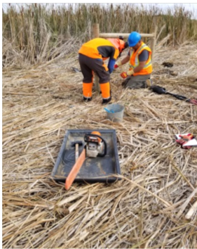
Sept 6/18 821 + 183.3 Photo taken facing east workers putting up the post for fence
