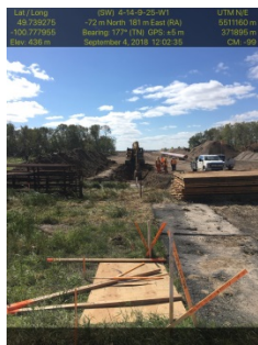
Sept 4/18 SSKP 824+350 Excavator digging exit hole on south side Orange stakes indicating bore alignment Rig mats to right used for hotline crossings Bore section in background
