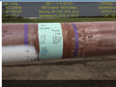
Sept 6/18 SSKP 826+475 – Facing north Coated weld after inspection Numbers indicate thickness Also did a V-cut to check integrity
