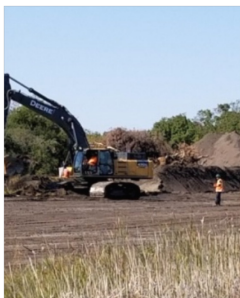
Sept 5/18 816 + 700 Excavator removing top soil and doing clearing Photo taken facing south
