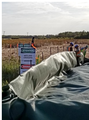
Sept 7/18 KP- 821+183.3 Photo facing east Workers laying geo tech Wetland Complex
