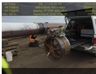
Sept 6/18 SSKP 825+400 Applus RTD- Testing with ultrasonic scanner Facing North
